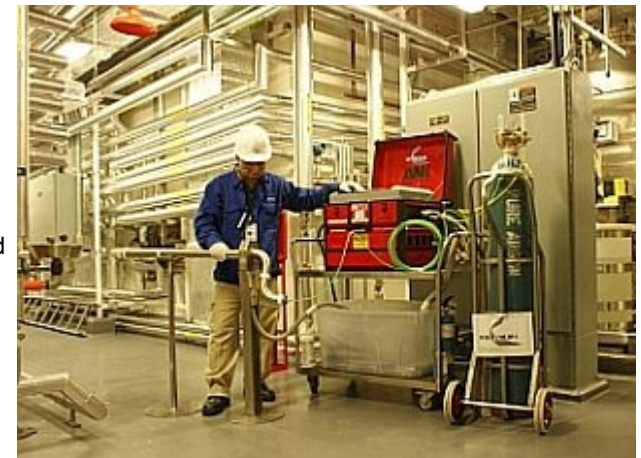
Figure 1. An orbital welding operator welding a tubing assembly at a biotechnology expansion in Singapore. Photo courtesy of Kenyon Engineering
